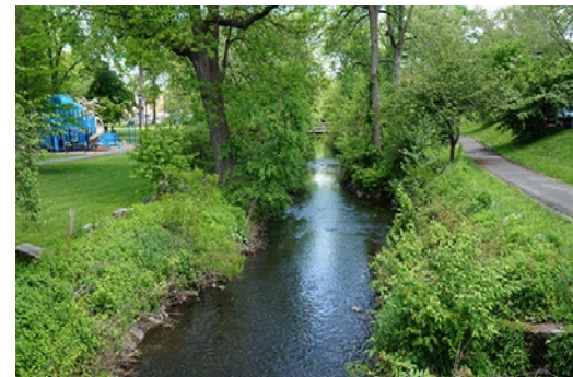
Figure 112: Results of a project to re-vegetate and stabilize the banks of the Sheldrake River in Columbus Park.
