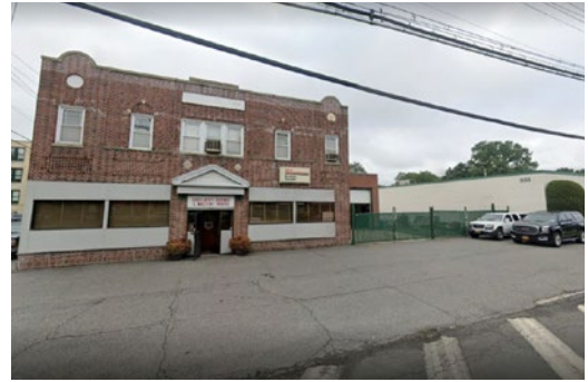
Figure 69: A wide expanse of asphalt fronts this building along Mamaroneck Avenue
