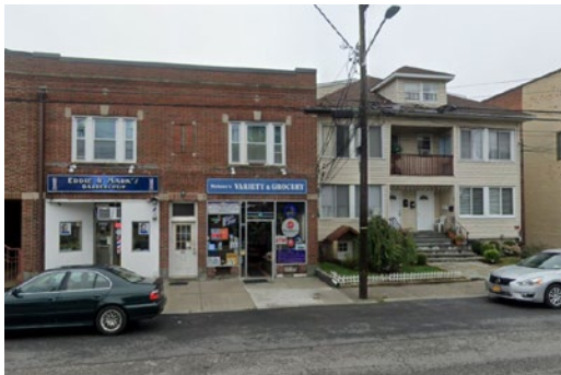
Figure 75: Several commercial storefronts and a two-family house located on Halstead Avenue
