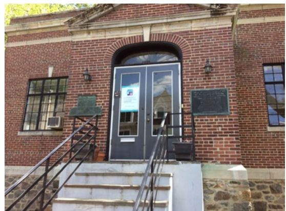
Figure 103: A historic building housing a counseling center has been undergoing renovations and is slated for further investment (photo courtesy of the Village of Mamaroneck)
