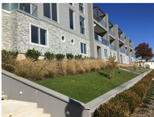
Figure 156: A new townhouse development along Post Road West utilizes green infrastructure, or vegetation to filter and absorb stormwater runoff.
