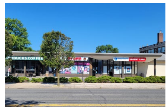
Figure 87: A commercial building on the 1000 block (north side) of Post Road West
