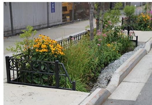
Figure 171: A bioswale, a type of green stormwater management technique, is designed to collect and absorb stormwater from the street before it enters the sewer system.
