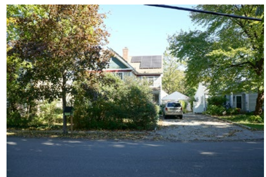
Figure 150: A house in the Village with solar panels on its roof.
