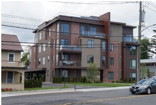
Figure 50: A recently-constructed apartment building along Post Road
