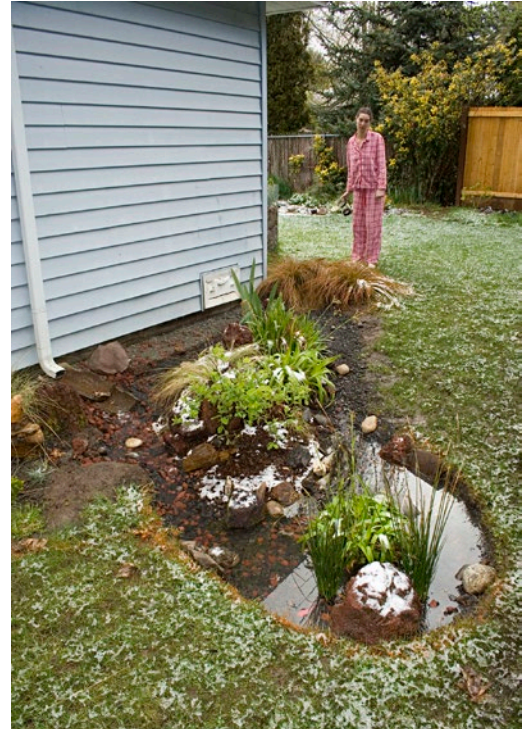
Figure 100: A rain garden created in a homeowner's yard collects rainwater from a downspout (photo by flickr user Beau Owerms, licensed under CC BY-NC-SA 2.0)
