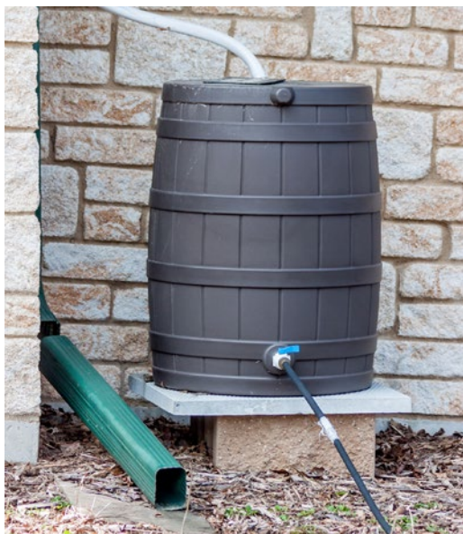
Figure 155: A rain barrel collects water from a roof of a house, which reduces stormwater runoff.
