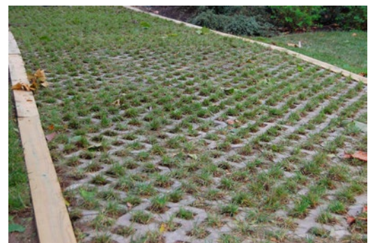
Figure 101: A driveway with a permeable surface (photo by flickr user Chesapeake Bay Program, licensed under CC BY-NC 2.0)
