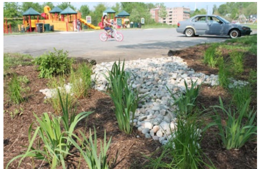
Figure 116: A rain garden collects runoff from a playground parking lot (photo by Elvert Barnes, licensed under CC BY-SA 2.0)
