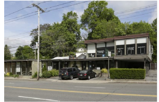
Figure 85: A commercial building on the 500 block (north side) of Post Road West
