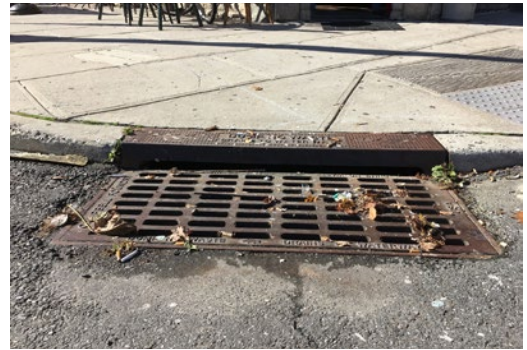
Figure 107: A storm drain
