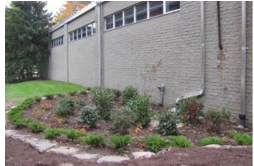
Figure 115: A rain garden collects runoff from the downspout of a municipal building (photo by Town of Mt. Pleasant)
