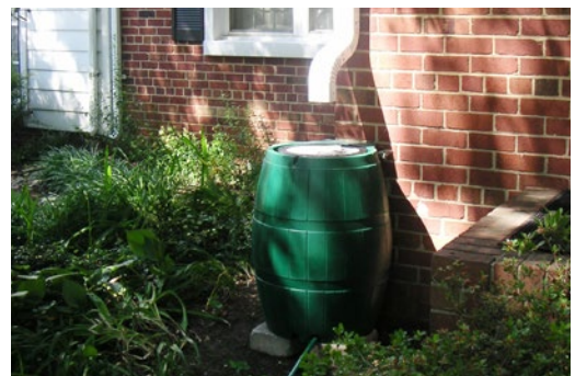
Figure 117: A rain barrel collects rainwater from the roof of a home (photo by Arlington County, VA)
