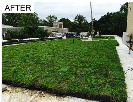
Figure 168: Before and after images of the Sarah Neuman Center's green roof.
