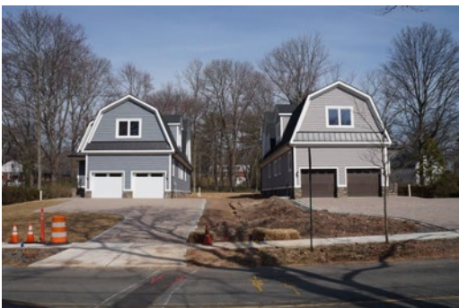
Figure 97: Two garage-first “snout-houses” in Princeton, NJ built after tearing down smaller houses.
